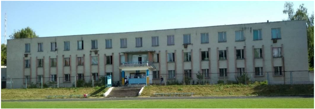
Fig. 4.2 – Panoramic view of the main facade of RO
